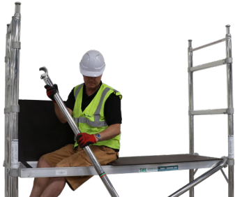
From a seated position descend down the tower to the next platform or ground. Ensure you always have collective protection around you when standing on any platform.
