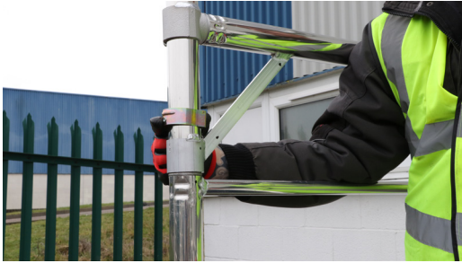
7. After adding frames always remember to engage interlock clips
