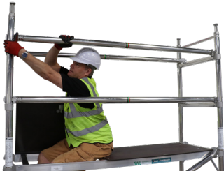
From a seated position remove 4 x guardrails making sure you never stand on an unprotected platform.
