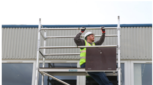
16. From a seated position, using the 3T method, fit 4 horizontal braces above the appropriate rungs to the frame vertices, hooks facing out.
