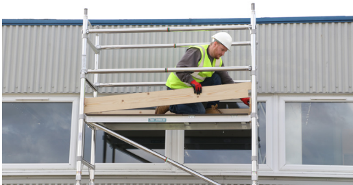
17. Fit toe-boards in correct position
