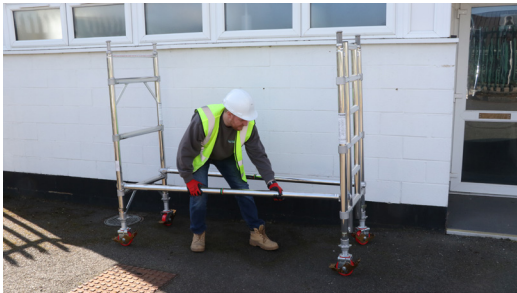
4. Fit 2 horizontal braces to the vertical member of the frames above first rung. Horizontal braces fit on from the inside of the tower facing outwards
