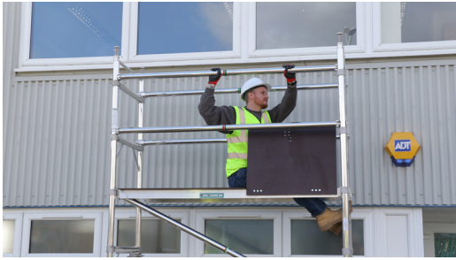
13. From a seated position using the through the trapdoor (3T) method. Fit 4 horizontal braces, hooks facing outwards to the frame upright.
