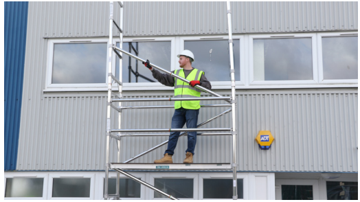
14. Continue erecting the tower fitting the frames and diagonal braces as illustrated using all components. Platforms inserted every 2m complete with handrails. Braces run in a continuous pattern on opposite sides.
