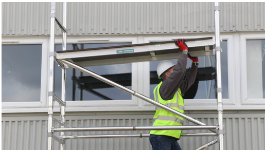
15. For your working platform fit trapdoor on the 3rd rung down from the top of the tower.
