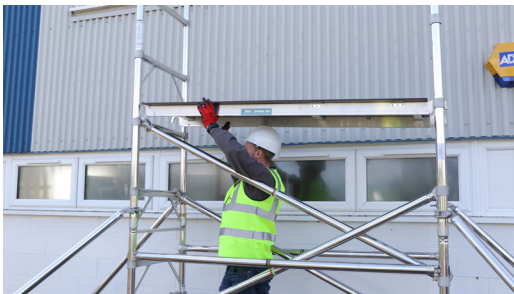
11. From the temporary platform, fit 1 diagonal brace to 3rd rung down and fit trapdoor platform over the hook. Offset platform to oneside.
